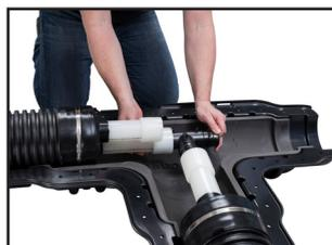
Push the expanded pipe end in quickly until it stops on the fitting nipple. Hold until the pipe has been shrunk.
